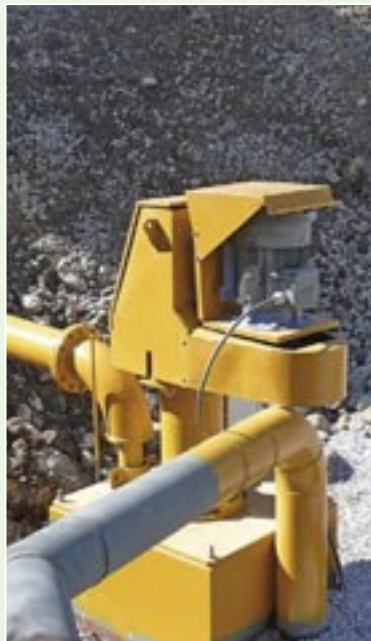
Pumpenstation Sumpf-Pumpe 100 RVHSP
